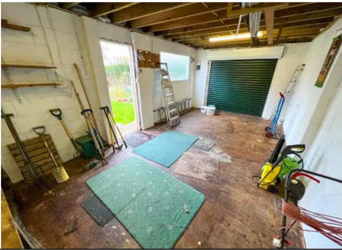
A photograph of inside the garage with power/light and electric roller door
