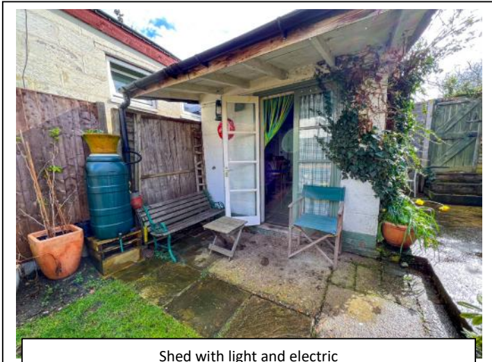
Shed with light and electric
