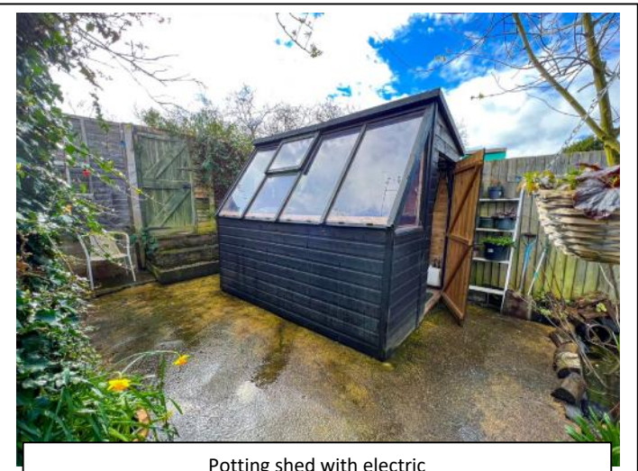
Potting shed with electric
