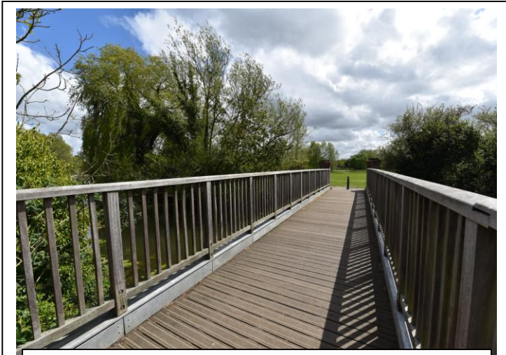
Bridge over the River Mole leading to Neilson Field
