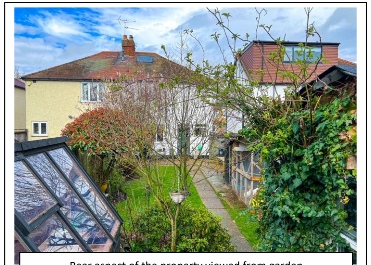
Rear aspect of the property viewed from garden
