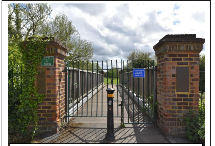
Gate to the pedestrian bridge leading to Neilson Field
