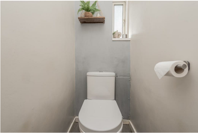
Double glazed window, low flush WC
