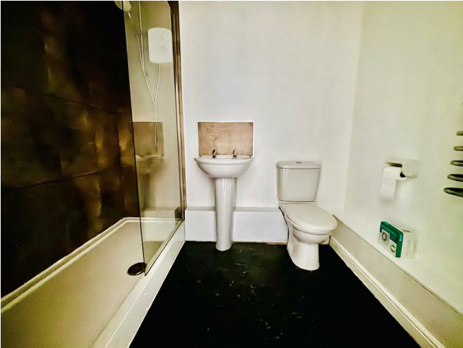
A suite comprising of a walk in shower with a glazed side screen & an electric shower above, low flush WC, wash basin, central heating radiator / towel warmer
